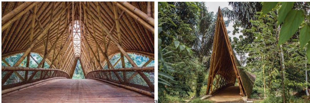
Figure 3. The Bamboo Bridge OUH
