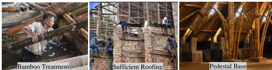
Figure 19. Three methods to enhance the bamboo durability
